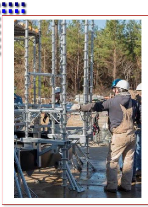
Starting Installation Of Excel Adjustable & Fixed Horizontals Into Excel Vertical Legs Assemblies
