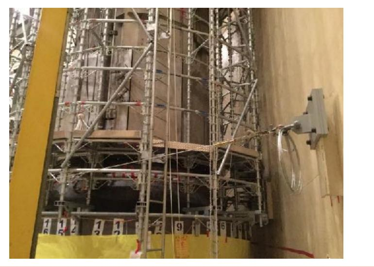
RVHFA Work Platform Sitting Next To Equipment Hatch With Reduced Footprint From Compact Design Allowed For More Efficient Move In Of Equipment Into <u>Ctmt</u>
