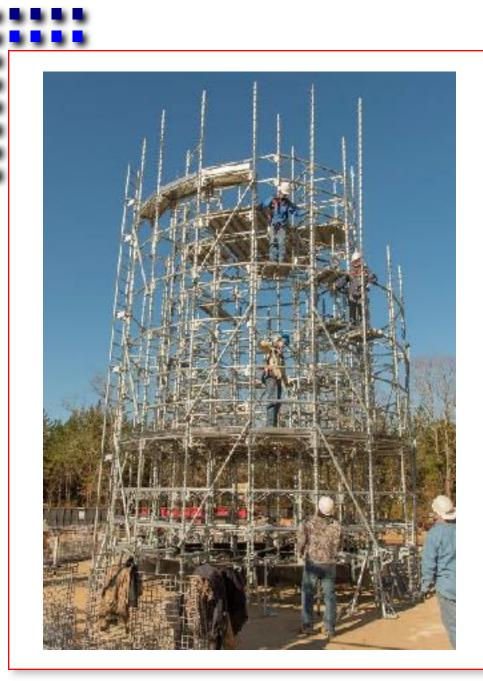
Installation Final Upper Wrap And Top Work Deck With Smaller Size Aluminum Deck Pans
