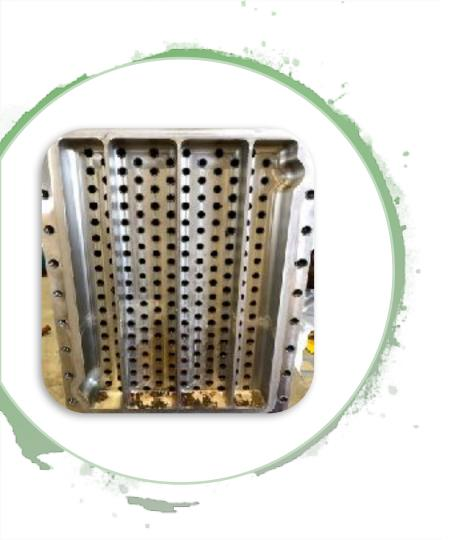
Callaway Plant Engineers wanted to find out how much sediment would be found on the outside of the tube sheet. This picture is typical of the material that was found when the head was separated from the sheet.
